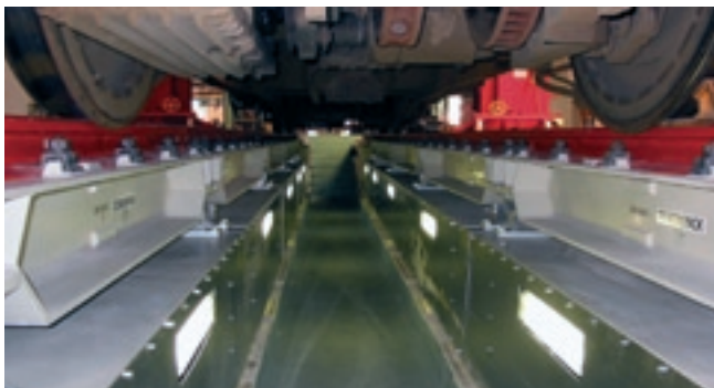
Figure 5: Accessible working pit
