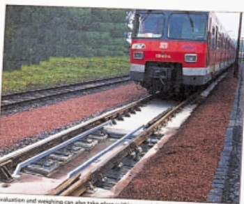
Evaluation and weighing can also take place within a specially constructed pit area
