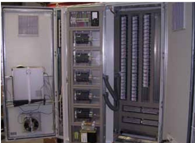
Fig. 18: Electronics cabinet for Y/Q measurement
